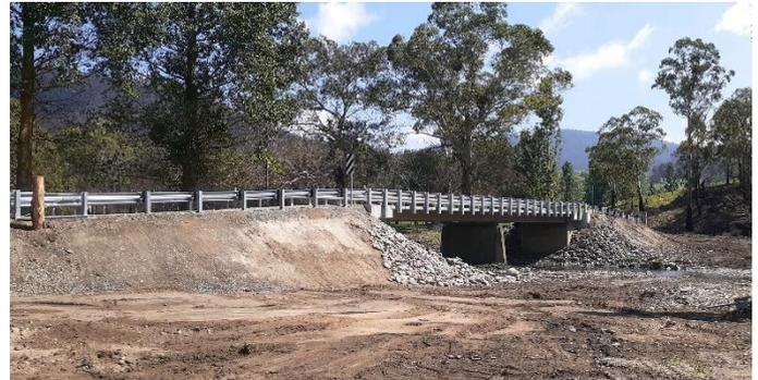
*We've completed, in partnership with our contractor, the upgrade of a fire damaged bridge on Timbarra River, Timbarra. The pre-cast concrete deck is 26 metres long and 4.6m wide. These bridge works were brought forward in our works program by about six months.*
