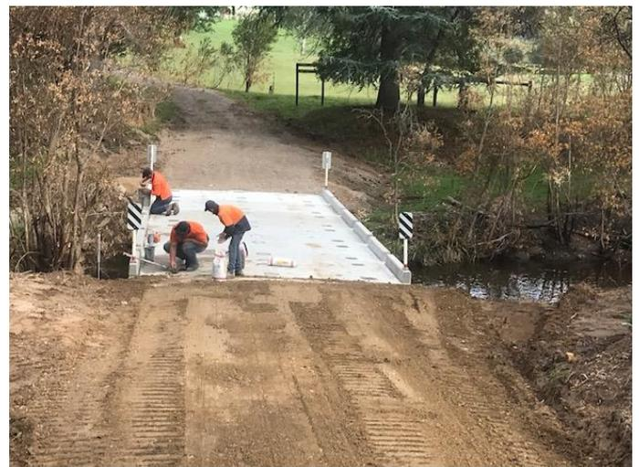
*Repairs to the bushfire-damaged bridge at Reeds Road, Goongerah, were completed last Friday. The timber deck was replaced with precast concrete panels, spanning 13 metres x 4.2m.*
