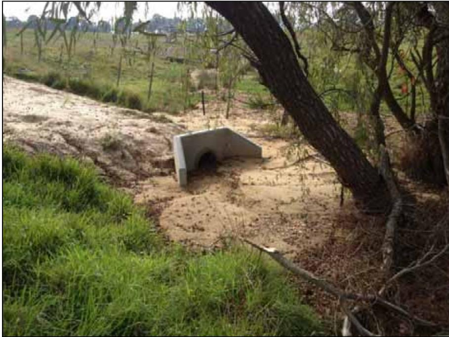
**Figure 4-5 Example of high sediment load to a natural waterway**
