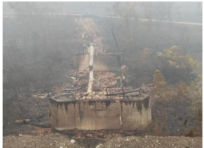
*Council has been able to inspect 16 bridges to date, with nine timber bridges destroyed or damaged beyond repair. Three are heritage listed. Four have been damaged but will be able to be repaired. We are anticipating a further six timber bridges have been destroyed. Above: Murrindal River Bridge, Buchan. Below: Waterholes Bridge, Deptford.*
